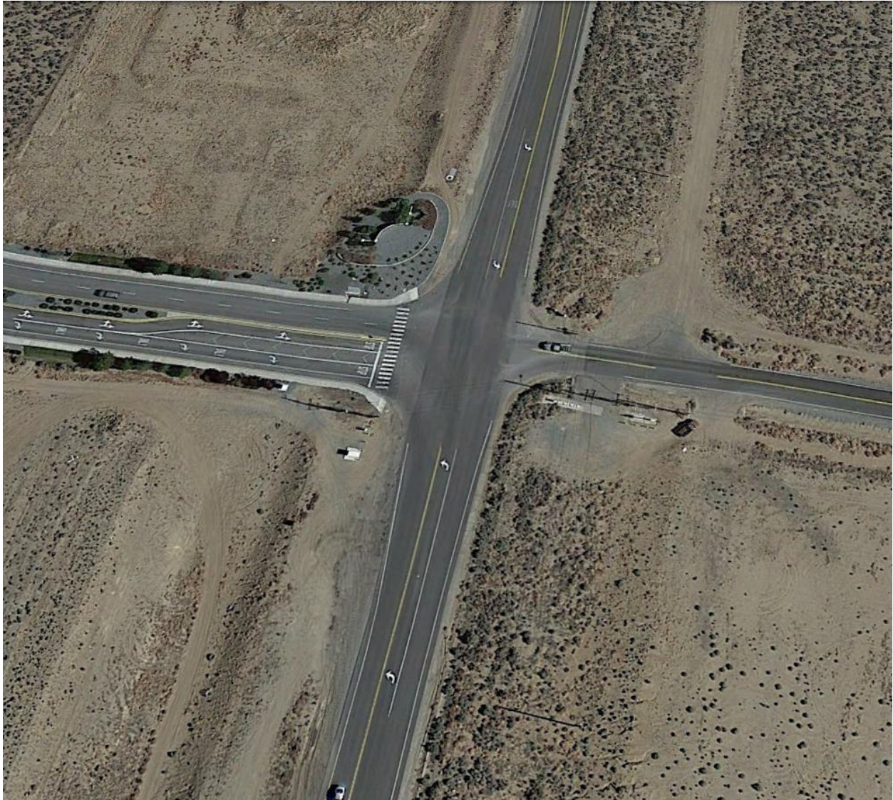
Exhibit II.D.4: Intersection Aerial and Photos
